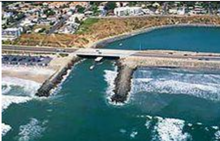
This one is a type of breakwater Jetty
