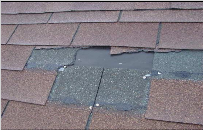
32-38 mph Shingles removed
